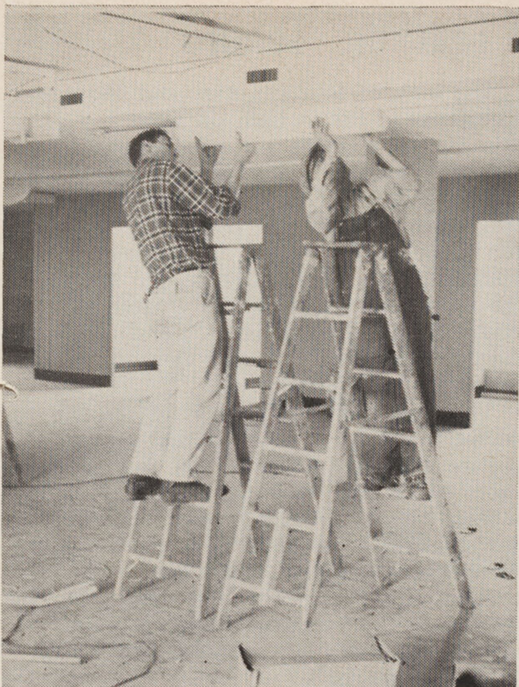
Interior work takes time.
