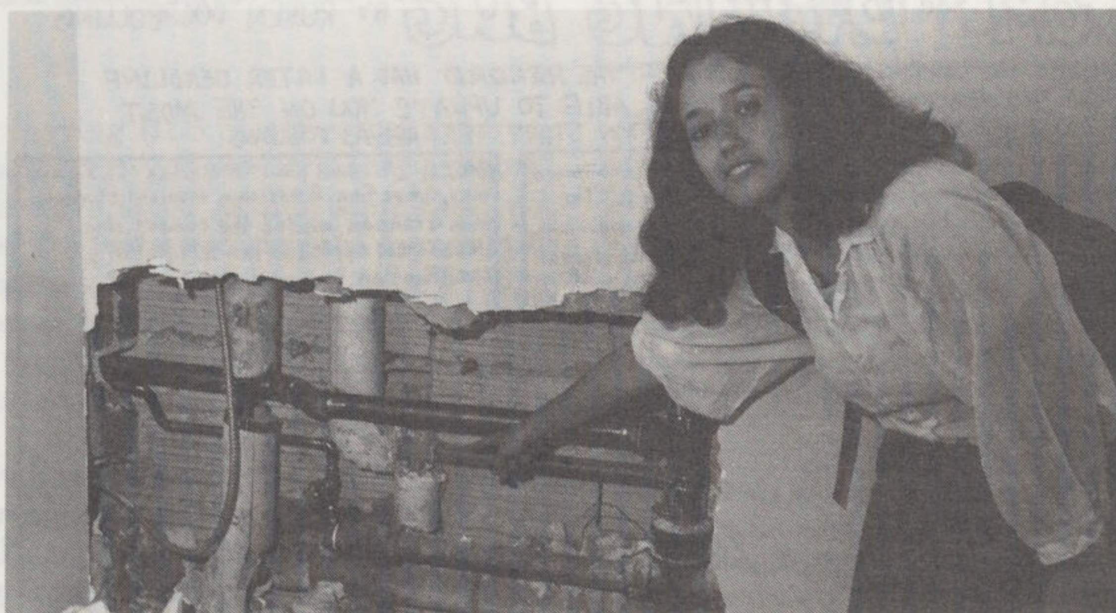
MBTA official points to service construction for new T-stop.
