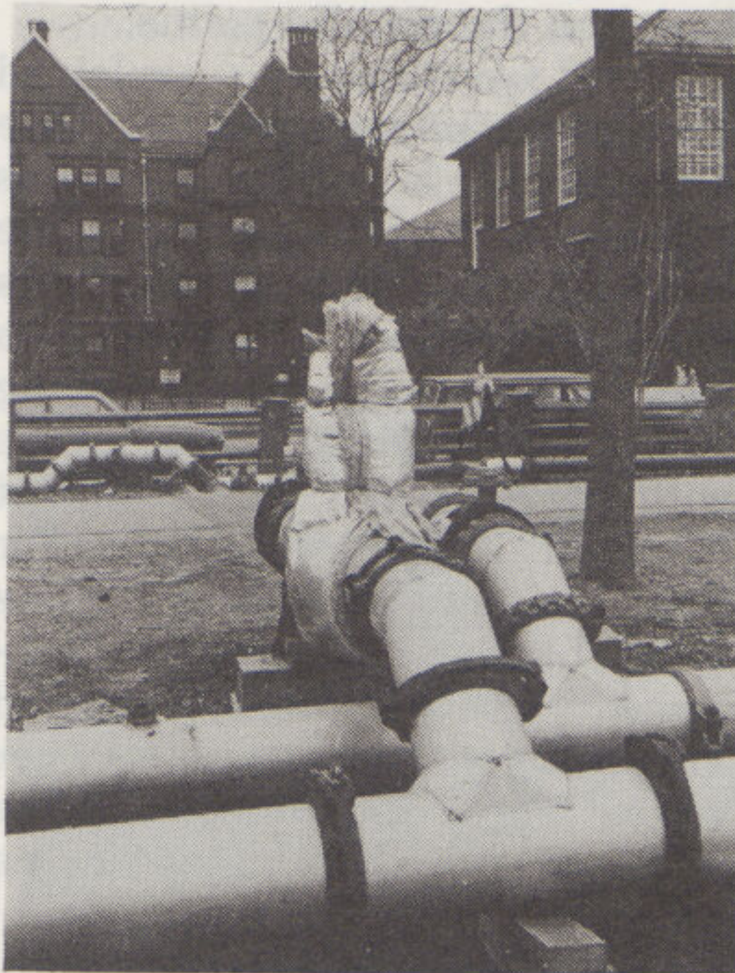
Pipelines that will soon carry the Law School's bounty to a Somerville generating plant.
