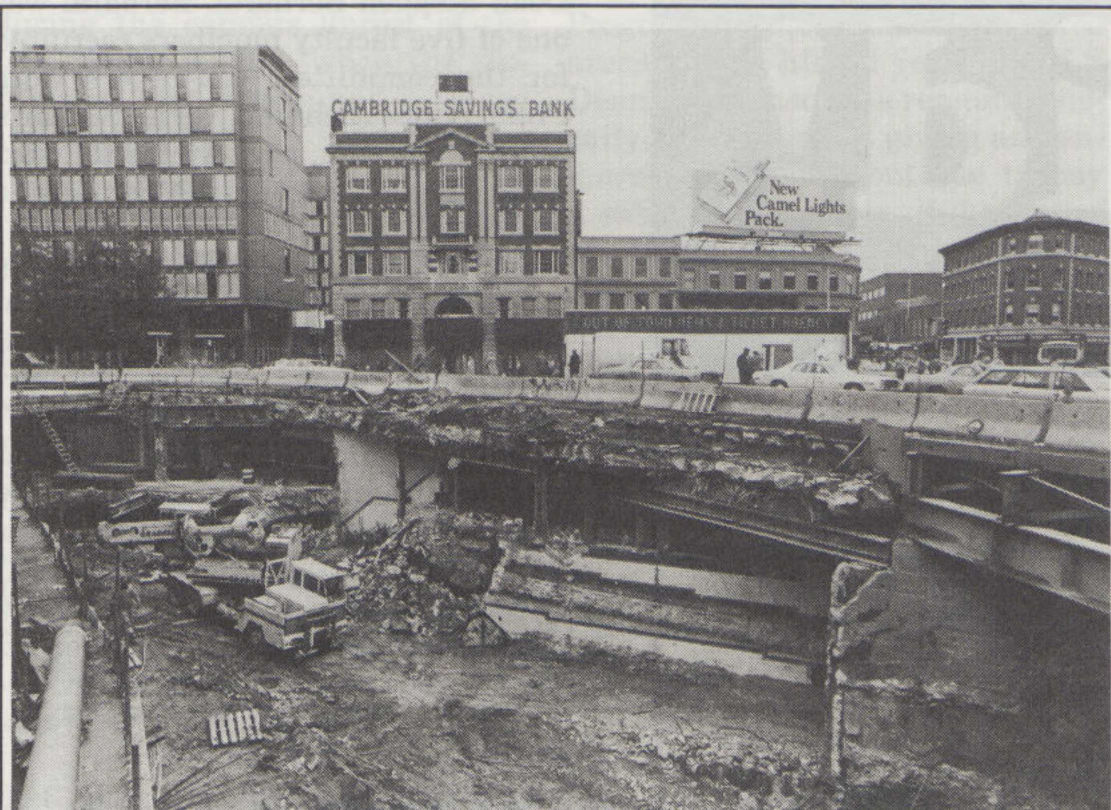
Demolition of the old Harvard Square T station continues. To the right in the lower portion of the picture can be seen the old bus tunnels which are being torn down to make way for the new Red Line tracks to Porter Square and Alewife. The bus tunnels are being rebuilt along with the new subway tunnel.
