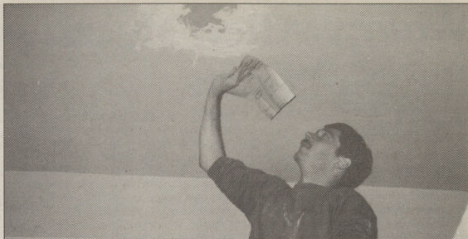
Michael Twomey '93 does repair work on Lincoln's Inn ceiling.
