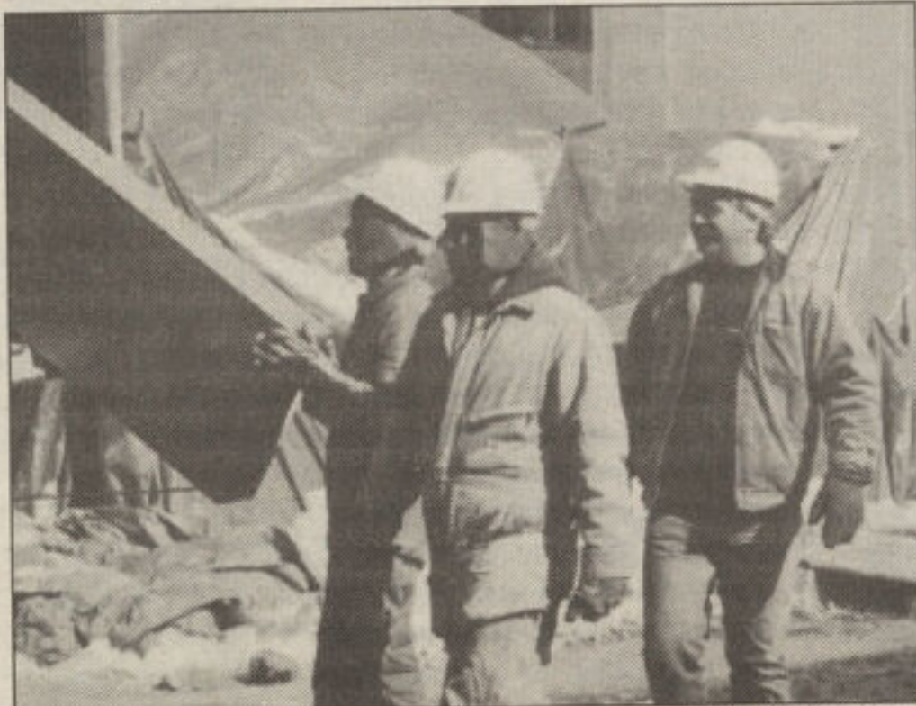
Holmes Field Building construction workers.
