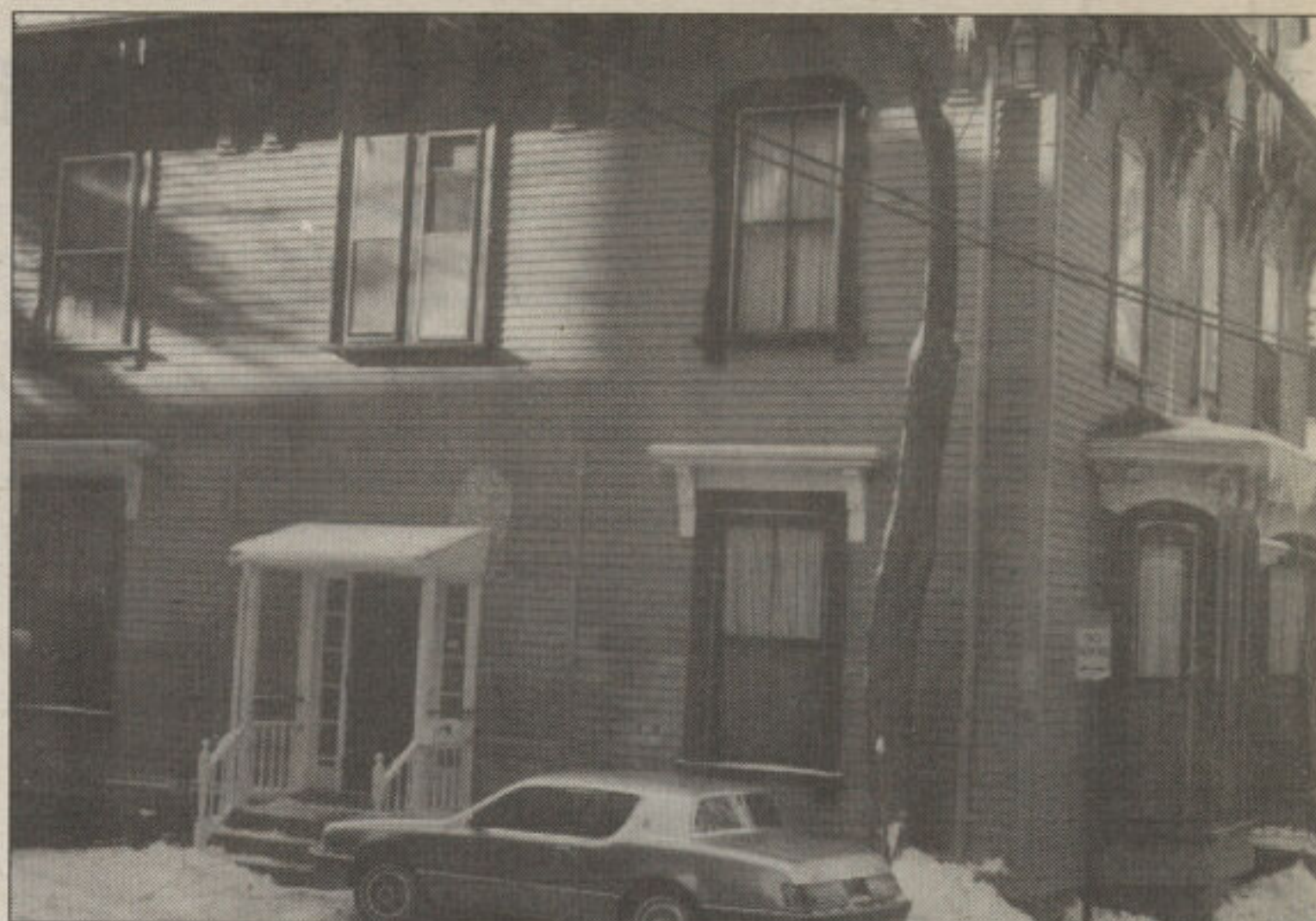
The Lincoln's Inn awaits a new paint job.
