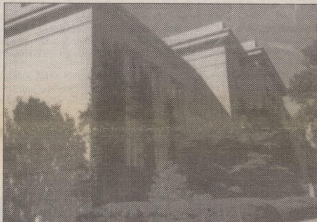
Langdell will receive its first major renovation since 1928.
