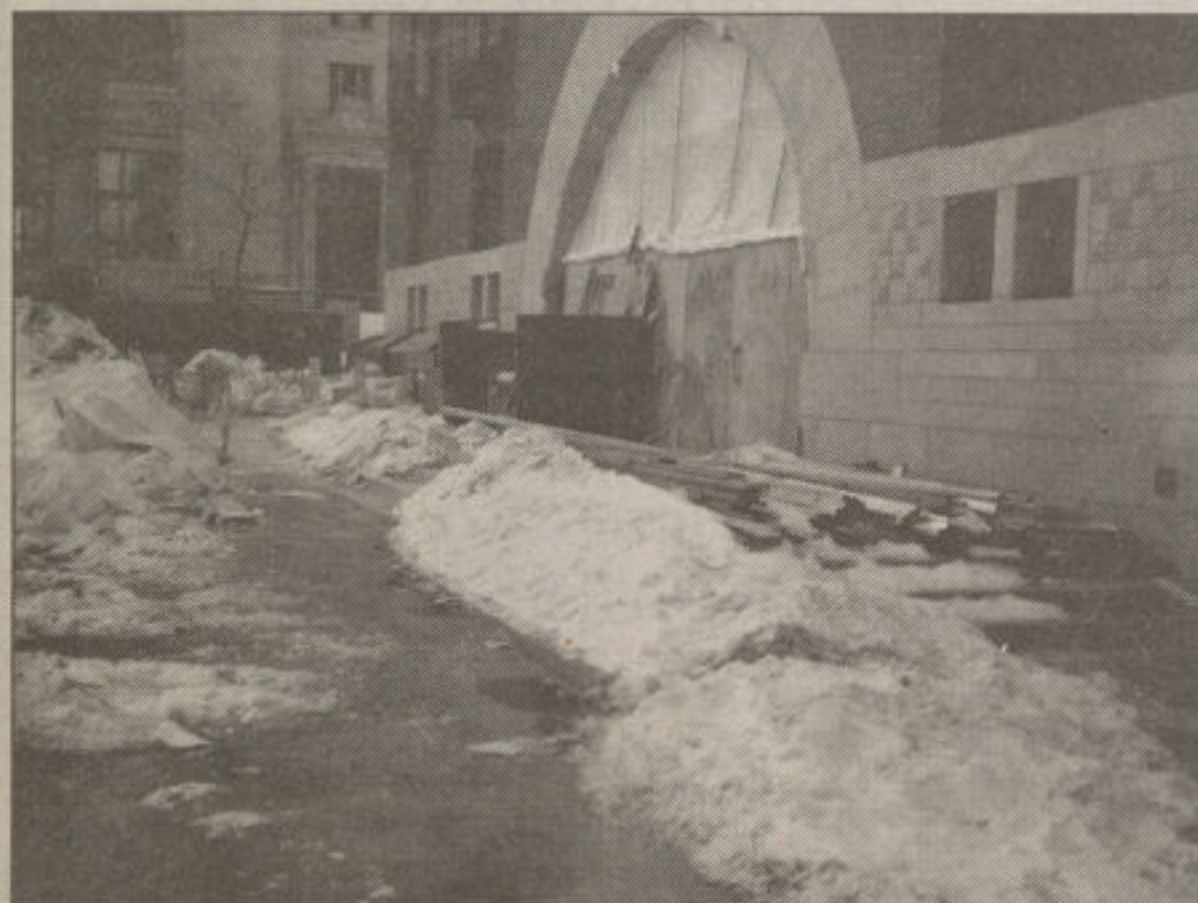
Entrance to the Holmes Field Building.
