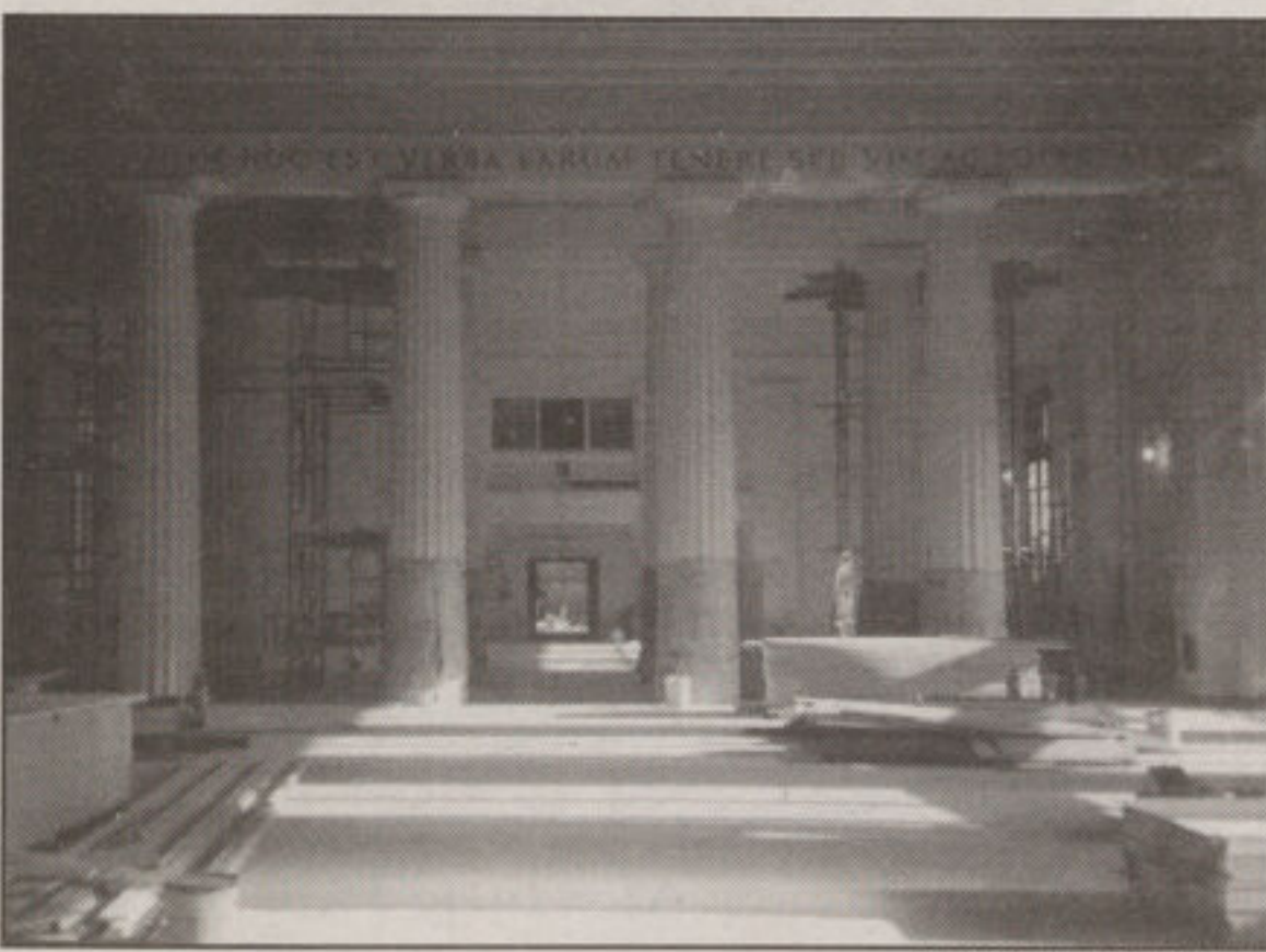
Langdell Library under construction
