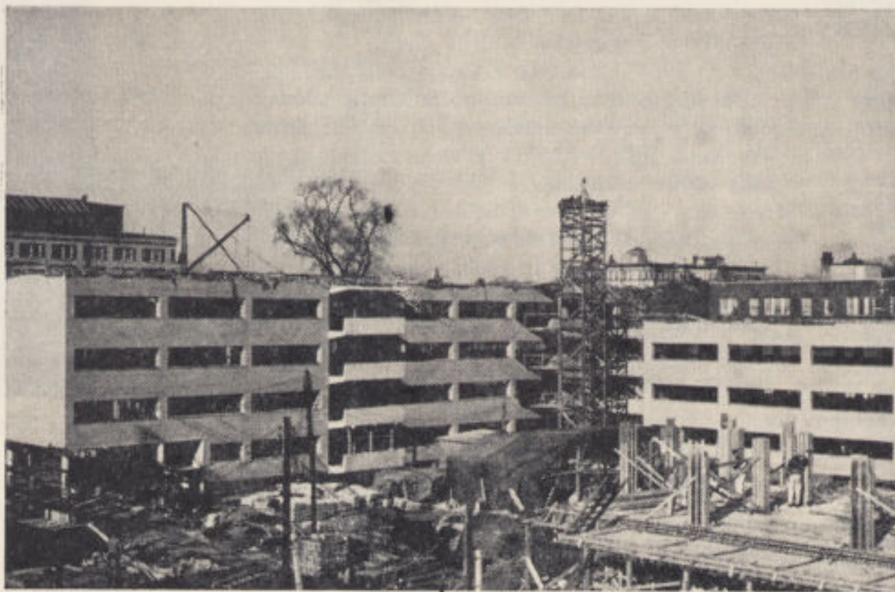
Pictured above are the new dormitories as the outside rapidly nears completion.
