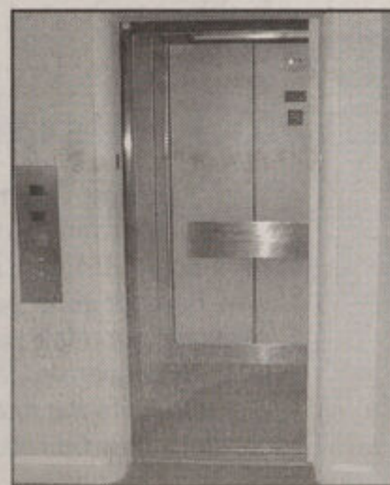
Inviting from the outside, these elevators are a tort waiting to happen.
