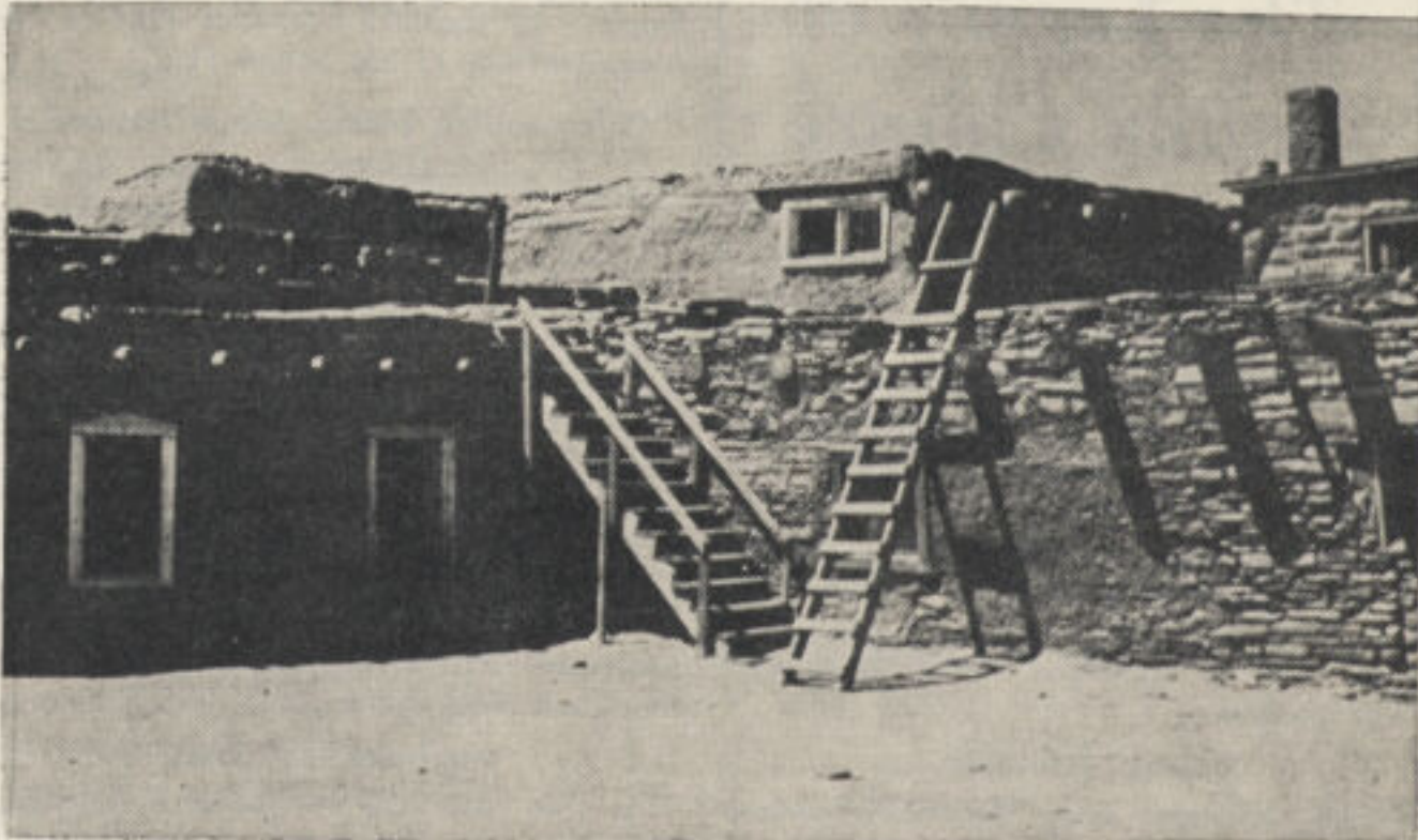
Two-story adobe pueblo helps to lessen the heat of the desert sun. The walls are 20 inches thick and are made of stone cemented and plastered with adobe mud. These terraced apartment houses are irregularly grouped into streets and plazas.
