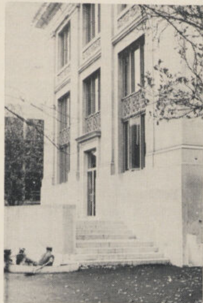
New Steps Leading into West Wing of Langdell Hall
